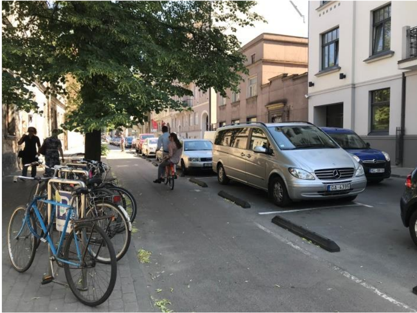
Figure 27. Cycle lane with light protection from motor vehicle traffic, Riga
